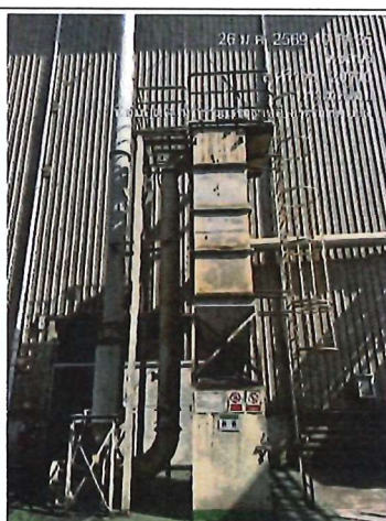
Dust Collector G.8 Forging 2
